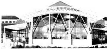
USAPT Headquarters bldg 3-3327 Butner rd.
